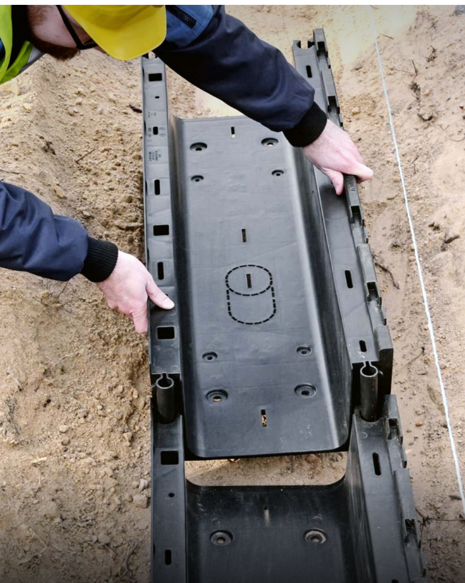
Fig. 1: Connecting of the cable ducts
