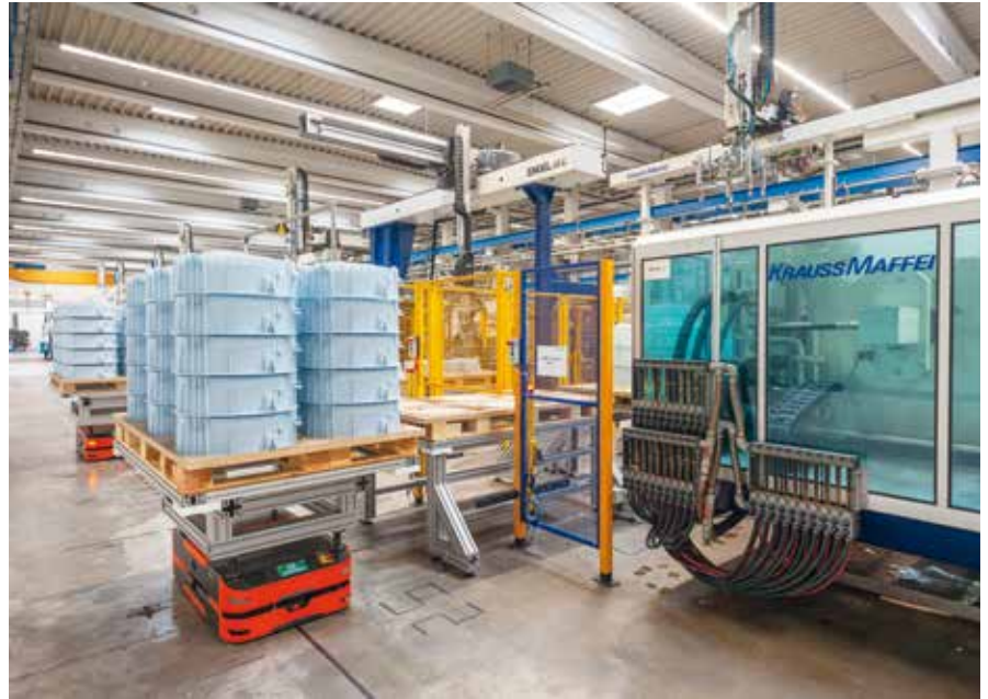
The supports for the linear robots on the various existing machines required several layouts in order to optimally arrange the pallet positions on each injection moulding machine.
