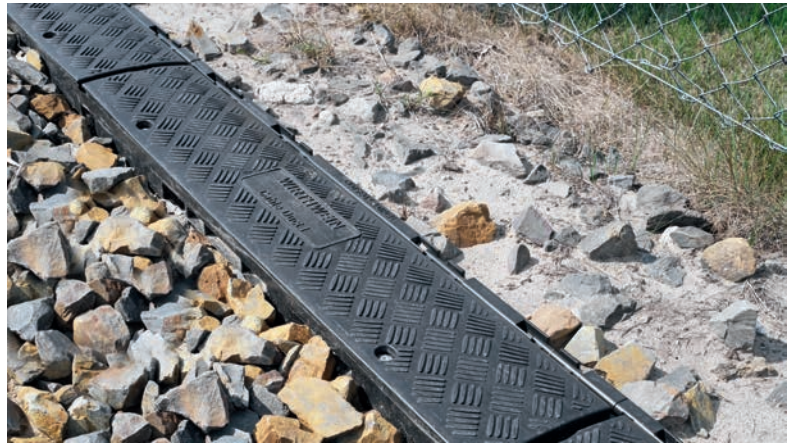
In modern railway lines, the plastic channels for energy and data lines are laid directly next to the track bed. © Wirthwein
